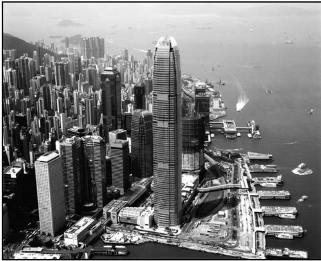
Figure 1. The Two IFC (International Finance Centre) Building
